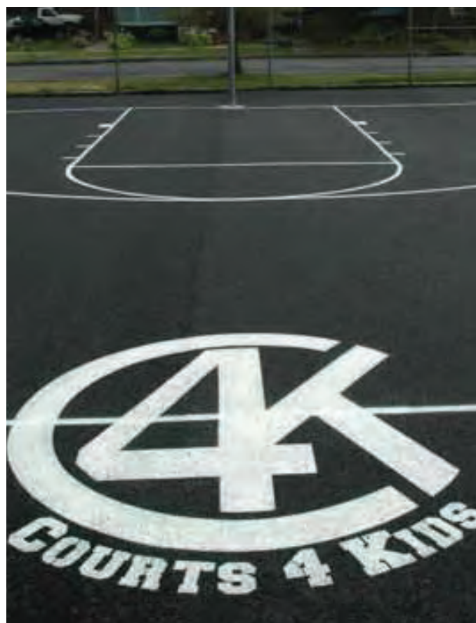
This porous basketball court minimizes stormwater runoff.
